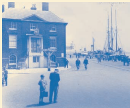
Custom House, July 1937; viewed from Harbour Office
