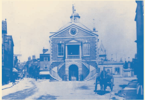
Market Street c.1900, looking towards the Guildhall and the police station
